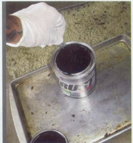
Never shake RustSeal; always stir, and stir thoroughly so material is "chunk-free." Also, never paint directly from the container.
